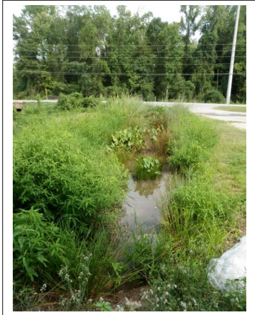
Figure 10. Wet Swale. (ACES, 2014, Alabama Low Impact Development Handbook)
